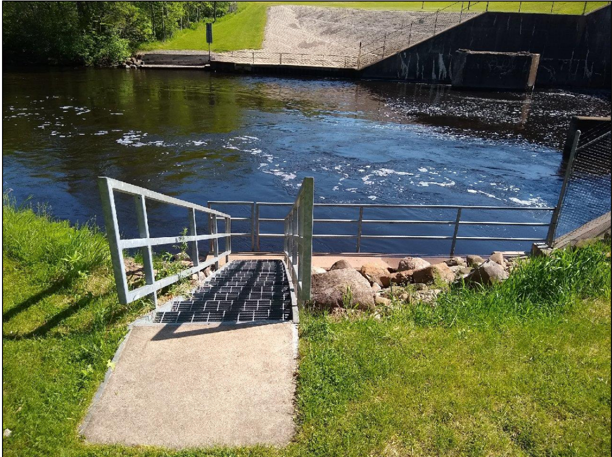
Figure 5.8.1.4.1-2 South Tailwater Access Stair and Fishing Area at the Trego Project
